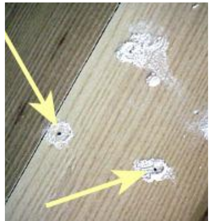
Powderpost damage of hardwood floors due to feeding. Note sawdust at entry holes.
